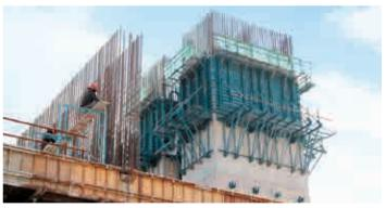
High early strength cement and concrete allow for faster formwork construction and removal
