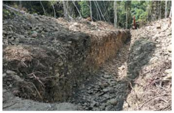
Drainage excavated to ensure constant flow with sufficient gravity-feed energy to power the micro hydro at Kampung Iburu, Sabah
