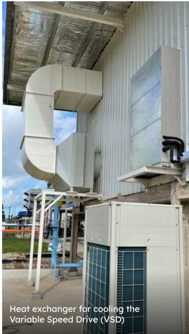
Heat exchanger for cooling the Variable Speed Drive (VSD)
