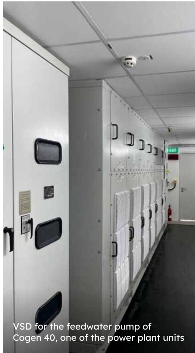
VSD for the feedwater pump of Cogen 40, one of the power plant units
