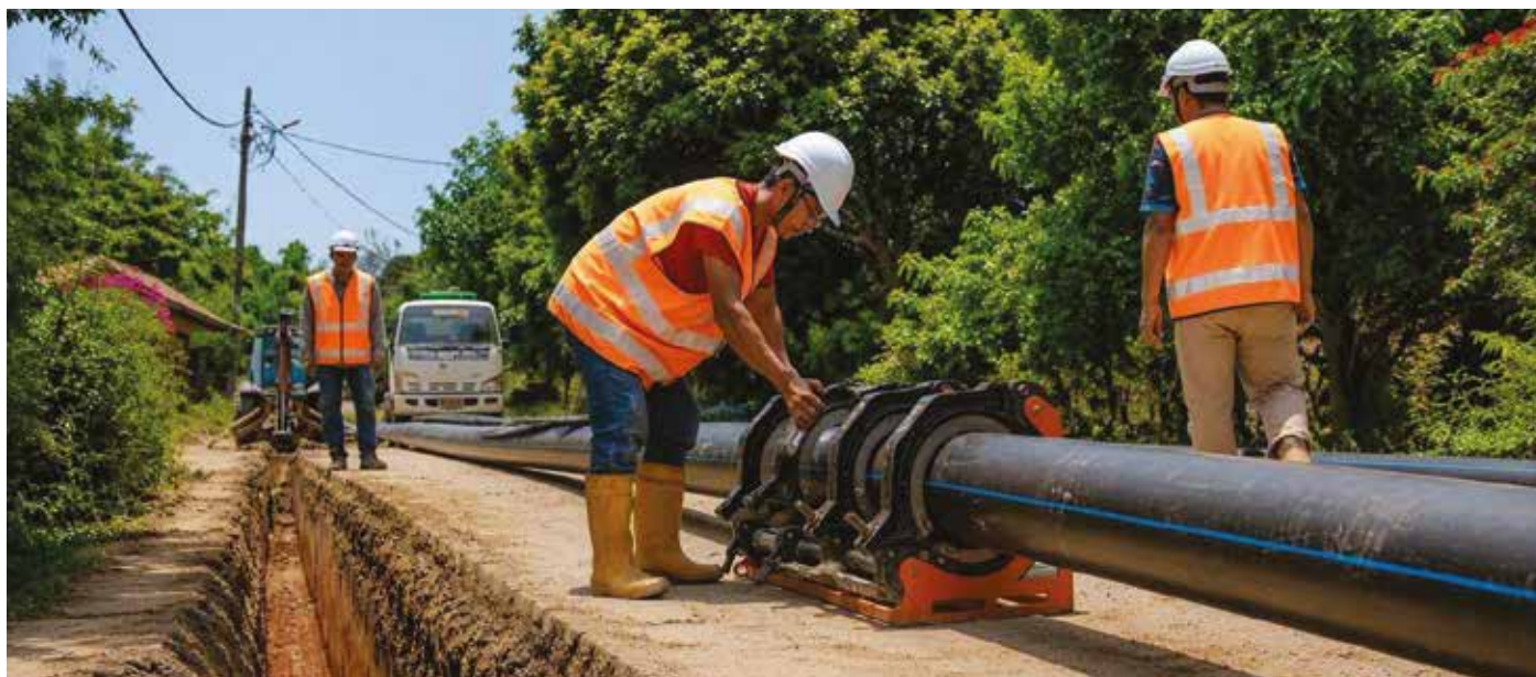
Pipe rehabilitation works undertaken to strengthen the distribution network, reduce water losses and improve the efficiency of treated water delivery to consumers.
