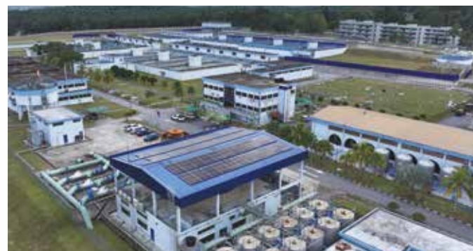
Ranhill's 63 kWp Solar PV System at 20 MLD, Sultan Iskandar
