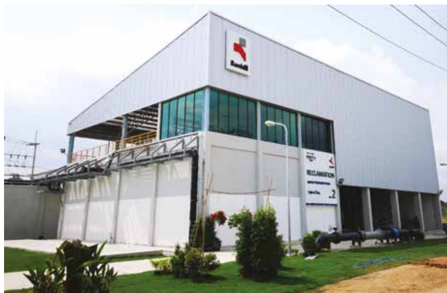
Reclamation Water Treatment Plant ("RWTP") at Amata City Industrial Estate, Rayong, Thailand.
